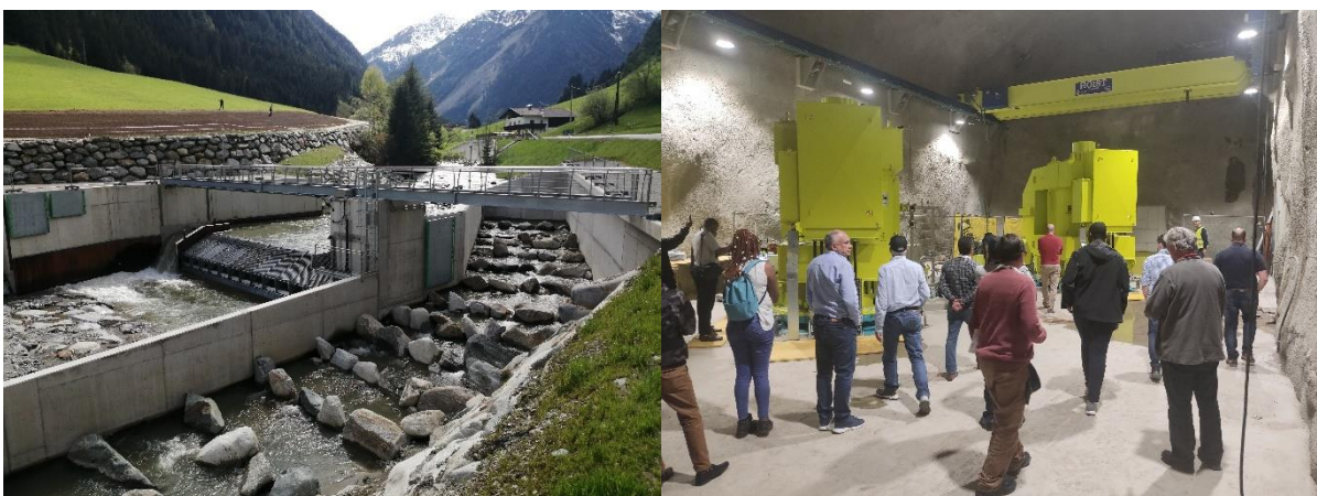
Figure 15: Site visit at Sellrain hydropower plant (on the left: general view of the hydropower plant intake, on the right: general view of the hydropower plant underground powerhouse)
