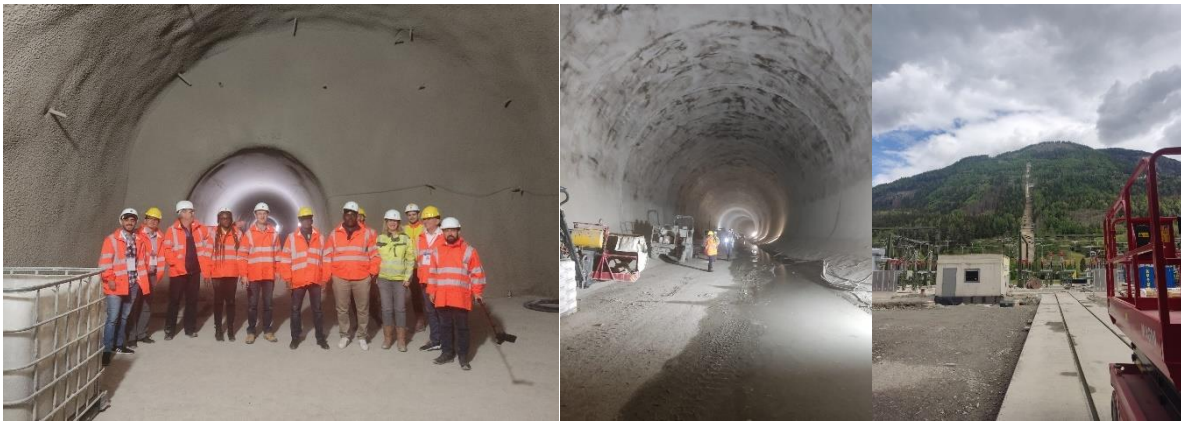
Figure 9: Site visit at Obervellach II hydropower plant (on the left: commemorative group photo at underground surge tank, in the middle: general view of the underground surge tank, on the right: general view of the hydropower plant penstock and transformer station)
