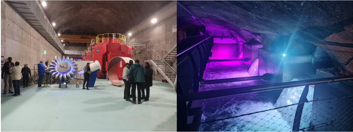
Figure 10: Site visit at St. Anton hydropower plant (on the left: general view of the hydropower plant underground powerhouse, on the right: general view of the underground surge tank)
