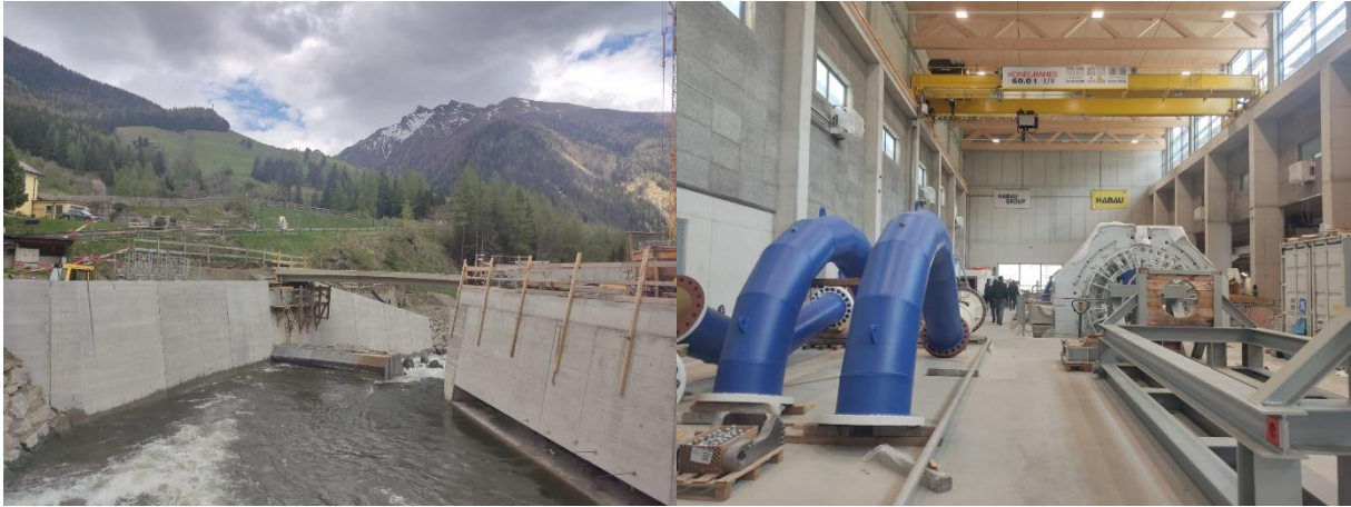
Figure 8: Site visit at Obervellach II hydropower plant (on the left: general view of the hydropower plant intake, on the right: general view of the hydropower plant powerhouse)
