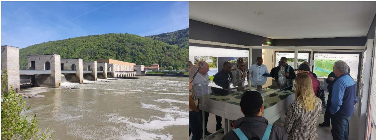
Figure 2: Site visit at Jochenstein hydropower plant (on the left: general view of the hydropower plant, on the right: participants at the visitor centre in the hydropower plant building)
