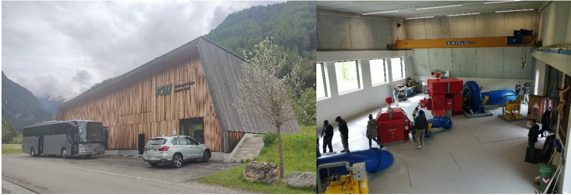
Figure 12: Site visit at Wiesen hydropower plant (on the left: general view of the hydropower plant powerhouse, on the right: inside view of the hydropower plant powerhouse)
