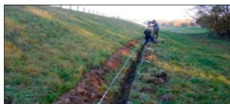
Fig. 7. Installation of the MPointS system, making only a shallow ditch to hide the cables. The cables may also be led through cable trays located on the ground.
