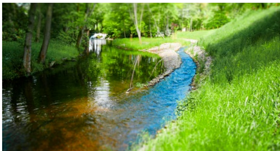
Photo 4. The removal of migration barrier on the Drawa River at Stary Młyn in Głęboczek within the Project: LIFE13 NAT/PL/000009 LIFEDRAVAPL. Bypass channel - a similar to natural stream fish pass while maintaining the riffle-pool sequence.ca River made within the framework of the Project: LIFE13 NAT/PL/000009 LIFEDRAVAPL in the area of the old weir between Jazwiny and Sówka.
