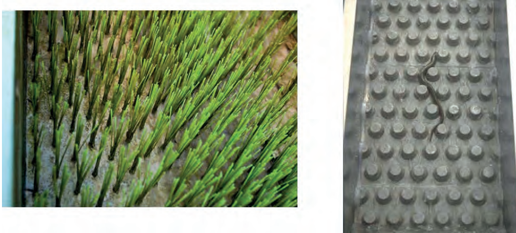
Figure 79: Eel ramp covered by a brush type substrate (left) and (right) a concrete cones substrate (source: AFB)
