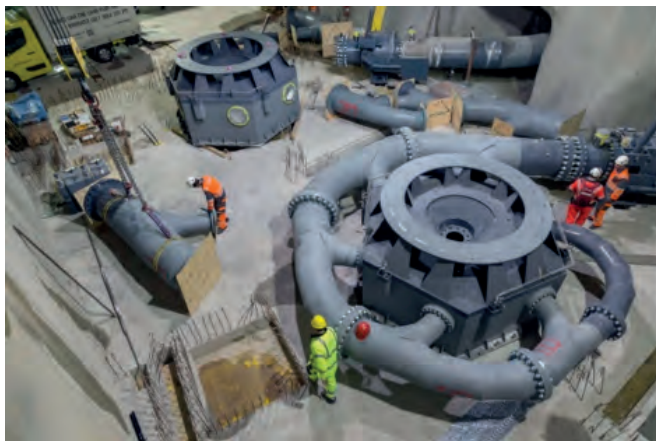
Figure 16: The 7 MW Pelton turbine of Gletsch Oberwald (CH) Hydropower plant (source: FMV SA)
