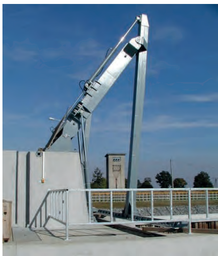
Figure 59: Articulated trash rack cleaner in Januszkowice SHP - Oder river, Poland (source: J. Steller)
