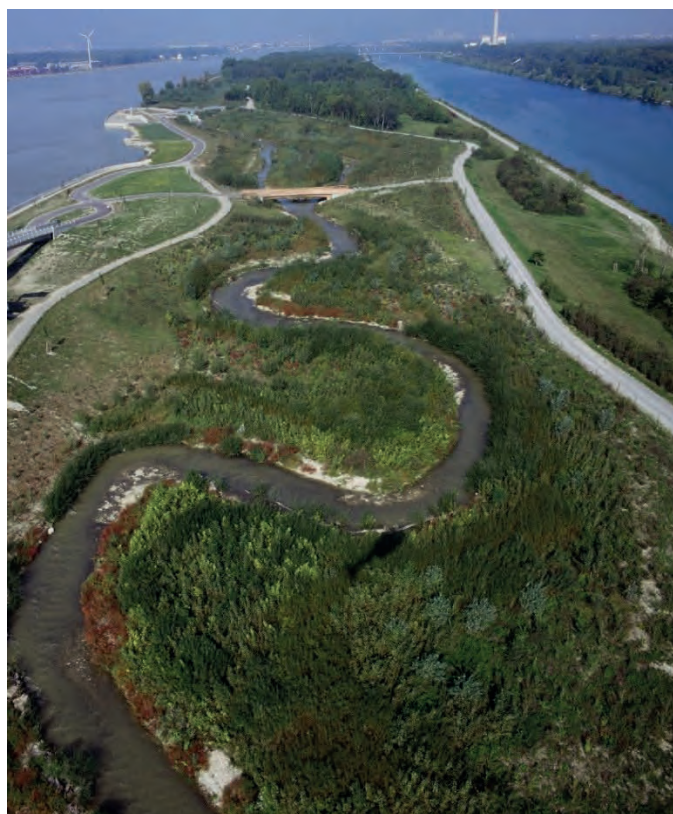
Figure 78: Nature like fishway at Freudenu HPP, Austria (source: W. Reckendorfer)
