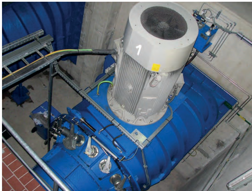
Figure 30: A typical compact unit with bevel speed increaser. Oborniki SHP, Poland (source: IMP PAN archives)
