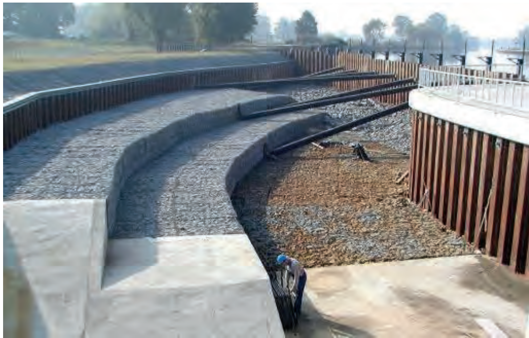
Figure 7: Shaping the inlet canal of Januszkowice SHP (1.5 MW) - Oder river, Poland (source: IMP PAN archives)
