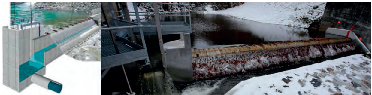
Figure 91: Coanda water intake illustration and example of Coanda water intake of Escouloubre (977 m altitude) on the Aude river, France (Source: AFB)
