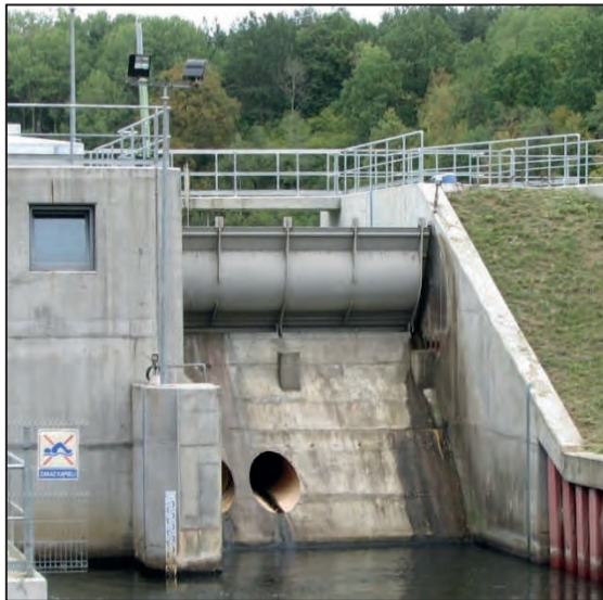
Figure 64: Weir crest hinged flap gate at Rzeczyca SHP - Wierzyca river, Poland (source: J. Steller)
