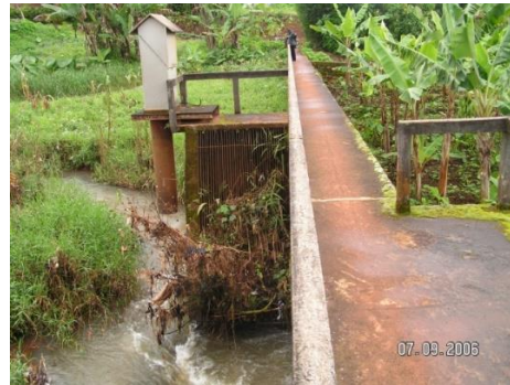
Fig. 7 Dam and intake of Dschang abandoned. microhydro plant
